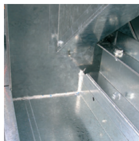
Watertight box in order to prevents condensate from escaping
