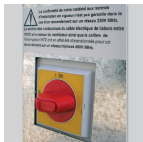
Start/stop switch mounted and wired
